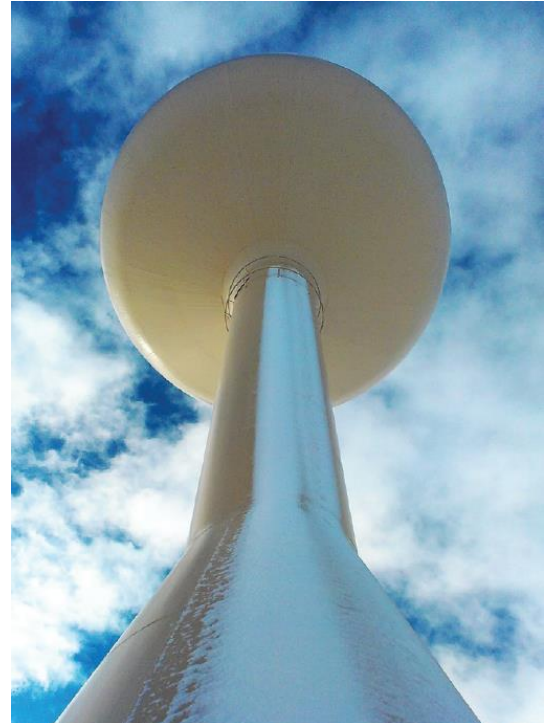
Figure 1. 300,000 gallon pedisphere in Laramie, WY. Winter temperatures are commonly below freezing for weeks at a time.
